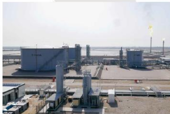
△ Central production facility
